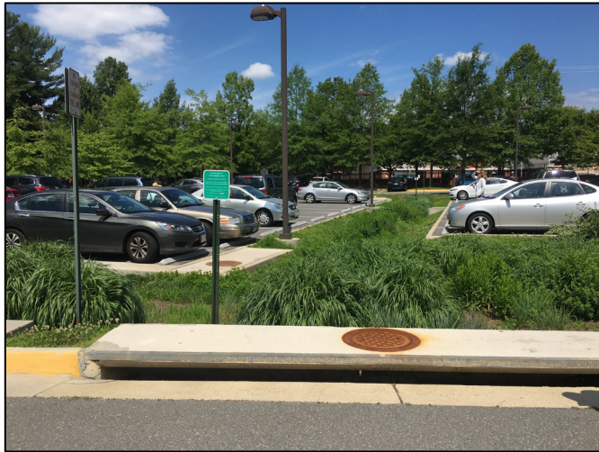
Photo, courtesy of Fairfax County, of a stormwater retrofit management practice.
