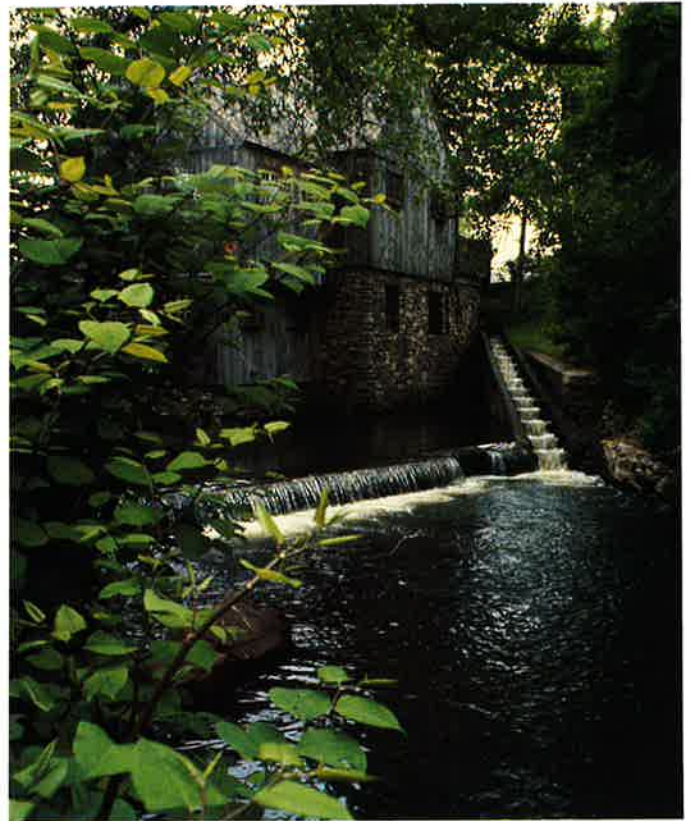
Historic mill dam with fish ladder. Small barrier dam directs fish toward base of ladder.
