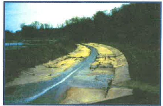
This urban stream channel has been drastically altered to increase stormwater drainage. Photo by Paul Kazzyak
