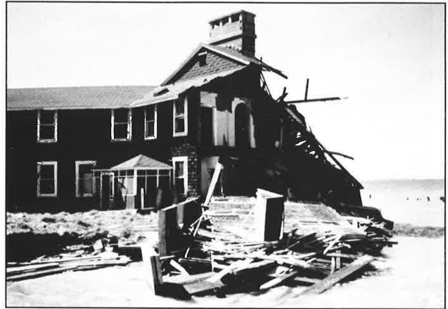
Figure 40. A hunting lodge on Barren Island collapses as shore erosion continues unabated (USFWS photo).
