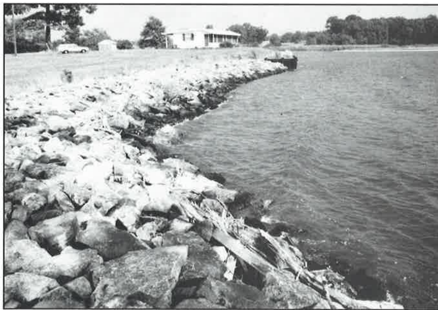
Figure 38. Riprap revetment is preferred over bulkheads for shore stabilization in the Bay (USFWS photo).
