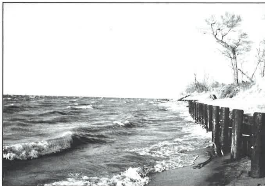
Figure 37. Bulkheads have been used extensively throughout the Bay to stabilize upland areas, but at the expense of the beach (USFWS photo).
