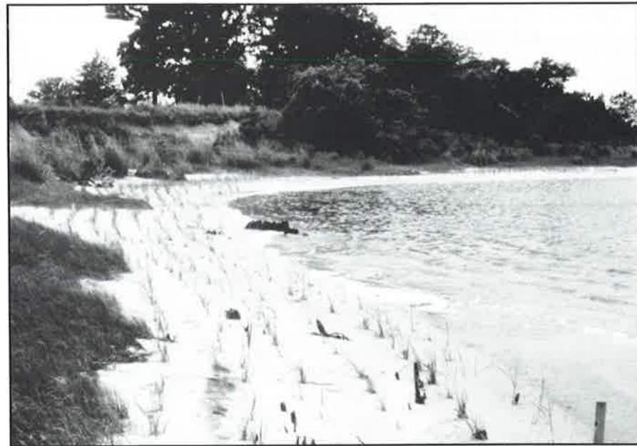
Figure 41. Marsh establishment is a nonstructural way to stabilize low-energy shores and provide habitat for fish and wildlife (top is planted area and bottom is same area a year later) (USFWS photos).
