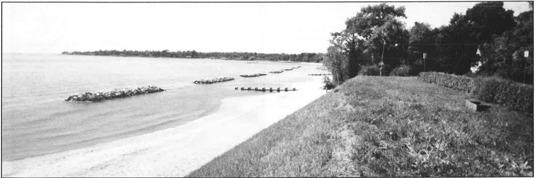
Figure 39. Offshore breakwaters with beach fill have been used at Bay Ridge, Annapolis to protect the cliff and provide a recreational beach (photo by Ed Fulford).
