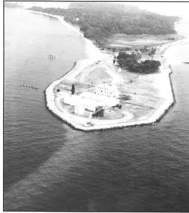
Figure 27. The Point Lookout Lighthouse area has been restored and stabilized but at the expense of the "point" (see Figure 26) (photo by Steven Leatherman).
