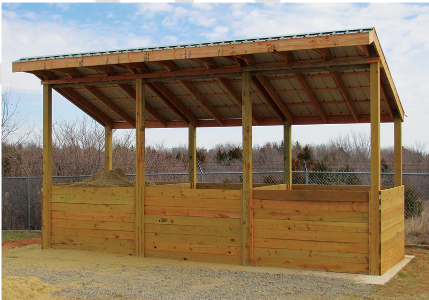
Figure II.3.4. "Three Bin" mortality composter (Langston University).
