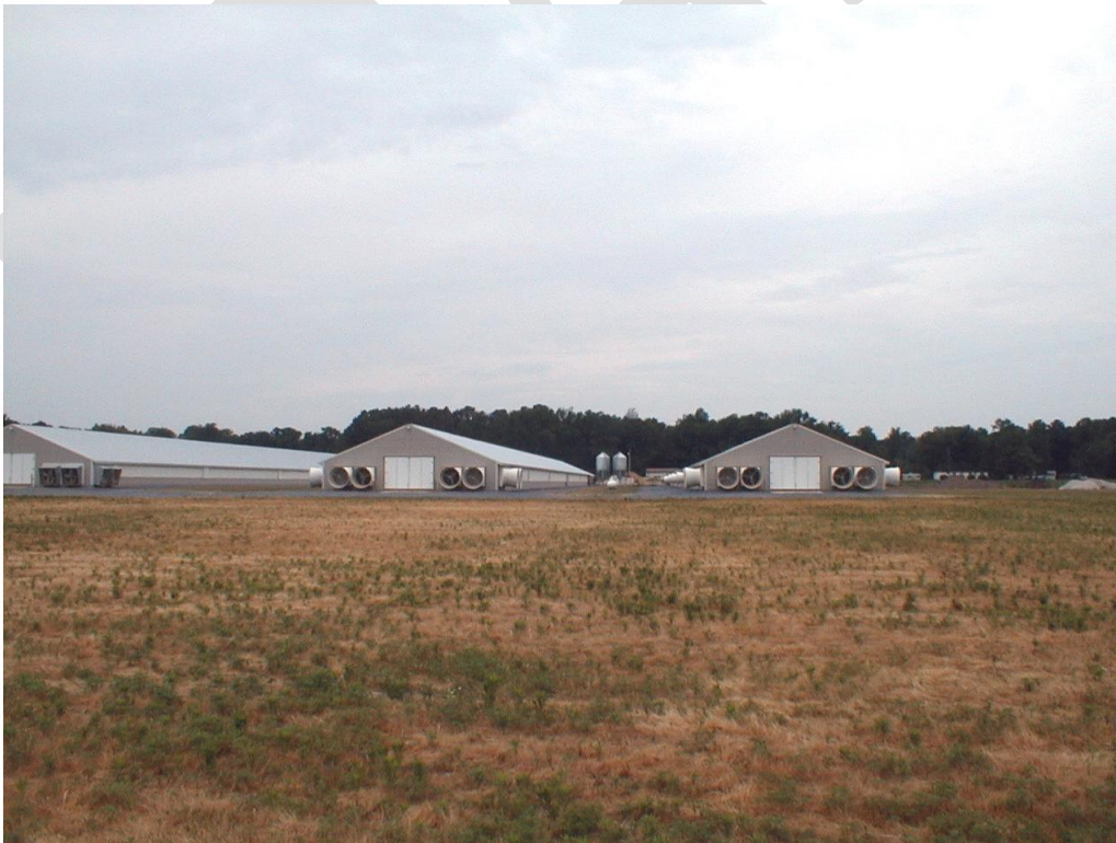
Figure I.2.2. Tunnel Ventilated Broiler Houses (Bud Malone).
