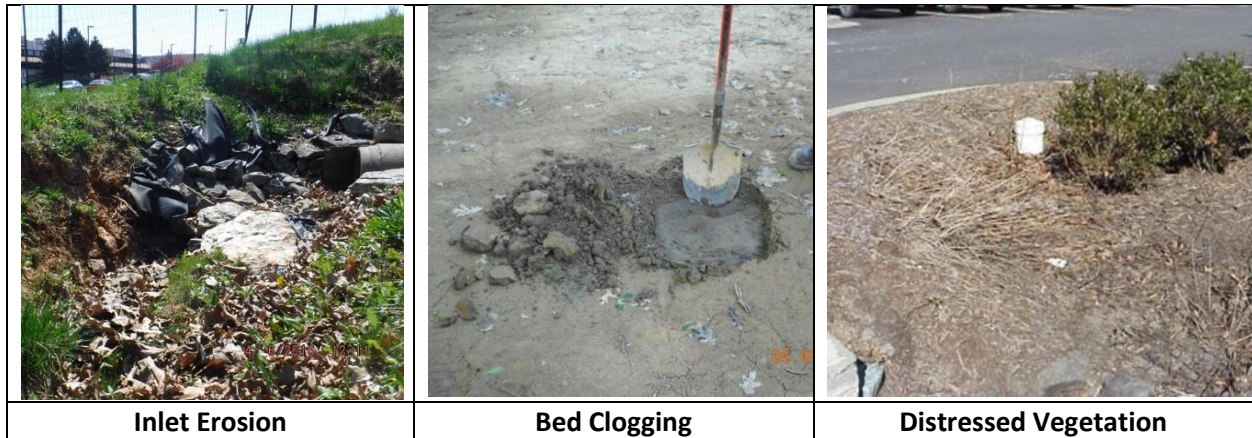
Figure 4. Examples of vulnerable design elements in upland LID practices.
