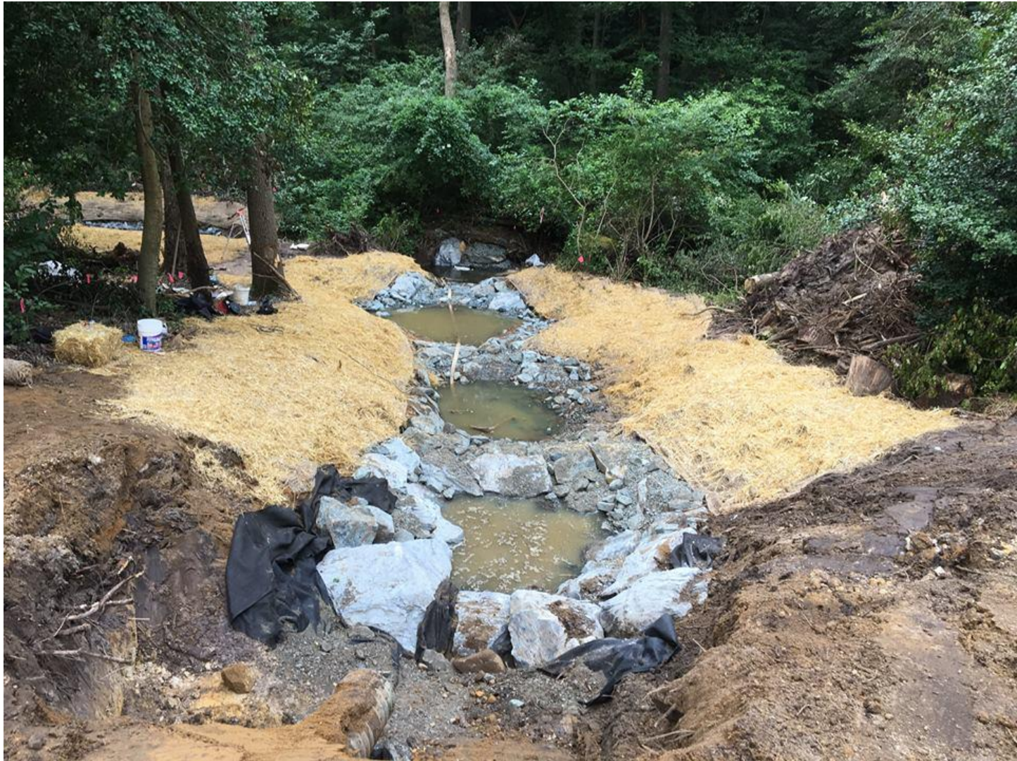
Stone step pools below outfall: courtesy Anne Arundel County DPW
