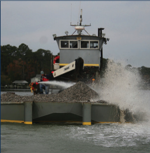
Contractors working for the U.S. Army Corps of Engineers, Norfolk District, use high-pressure water cannons to spread fossilized oyster shell in the Lynnhaven River in Virginia Beach, Va., in an effort to build medium relief oyster reefs for an ongoing oyster restoration project. (Photo courtesy USACE Norfolk)
