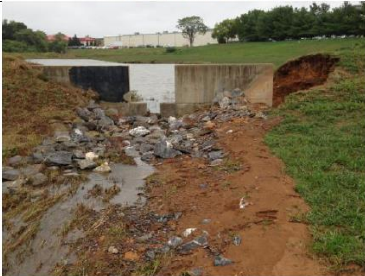
Embankment Failure
