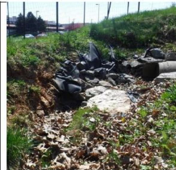
Inlet Erosion
