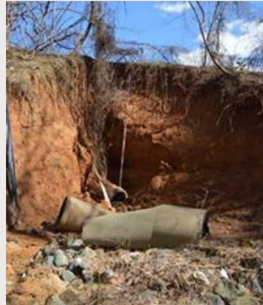
Figure 2.5: Stages of stormwater drainage failure due to sea-level rise. Graphic by Emily Niederman, Stetson University.
