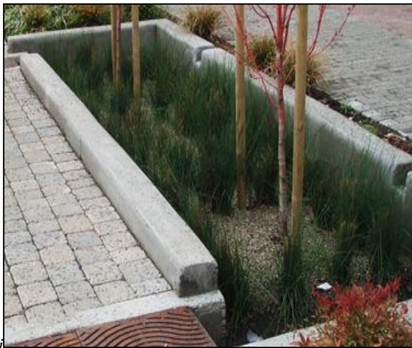
Figure 7 – Typical planter box (Source: Philadelphia Water Department, 2014)
