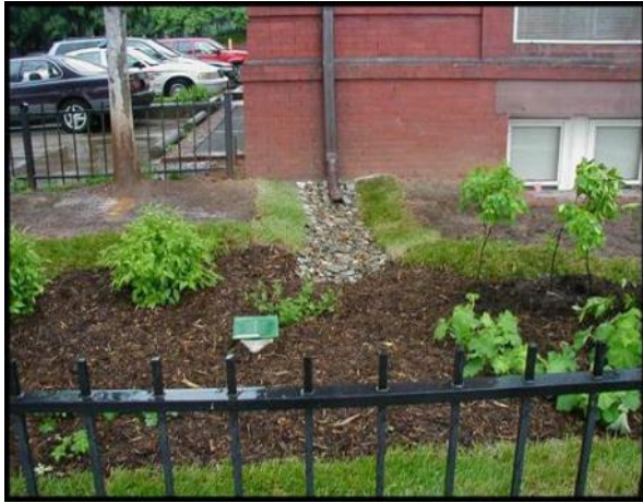
Figure 4 – Typical downspout disconnection configuration (Source: LID Center, 2005)
