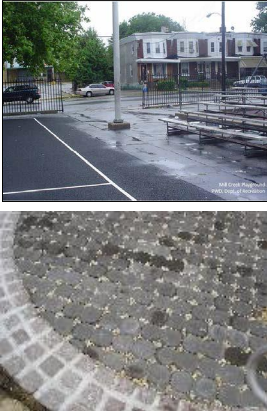
Figure 9 – Typical porous asphalt (top) and permeable paver (bottom) applications (Source: Philadelphia Water Department, 2012)
