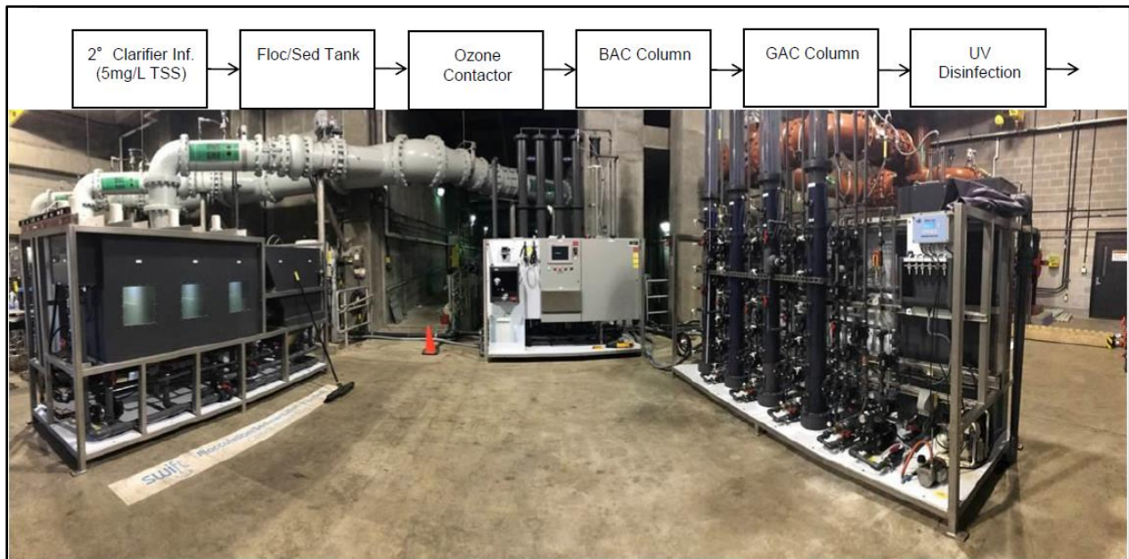
Figure 7. Diagram of HRSD Sustainable Water Initiative for Tomorrow (SWIFT) tertiary treatment train being utilized at the York River WWTP in Seaford, VA (HRSD 2019).
