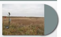
A view of an installed biomactor, showing the upper control structure and warm season grosses that have re-established in soil covering the bed of wood chips in which water is meeted.
