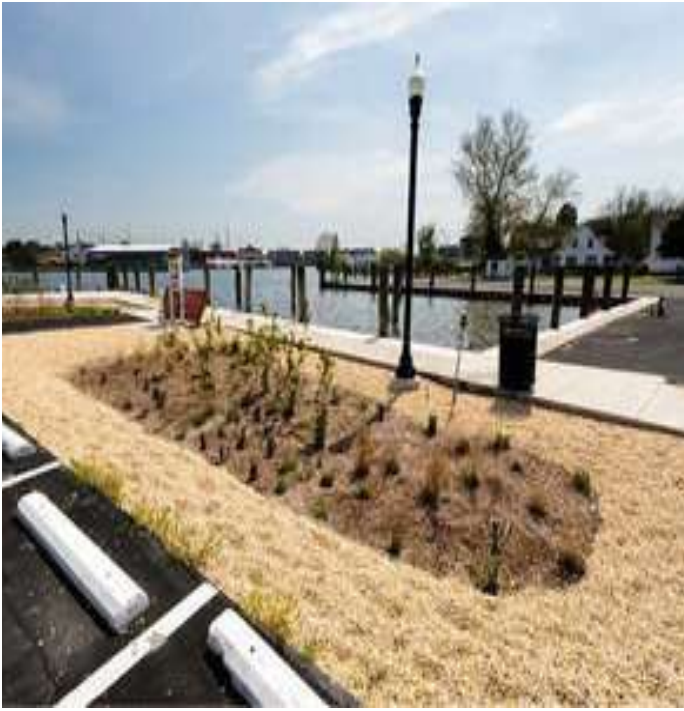
A rain garden at Long Wharf Park captures and filters storm water pollution before it reaches the Choptank River in Cambridge, MD. Photo by Will Parson/Chesapeake Bay Program
