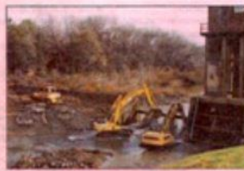
Courtesy of Restoration Systems The old dam near Carbondon in Chatham County was removed in early 2006. The site had hosted several dams throughout the 17th century.
